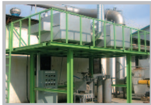
▼ 촉매연소열교환기 (Catalytic Combustor with Heat Exchanger)
